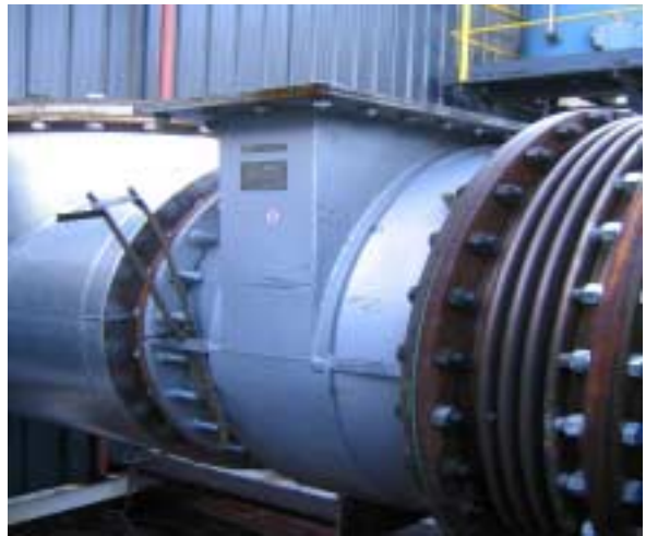
Figure 4: DCL QUICK-LID™ catalyst reactor housing
