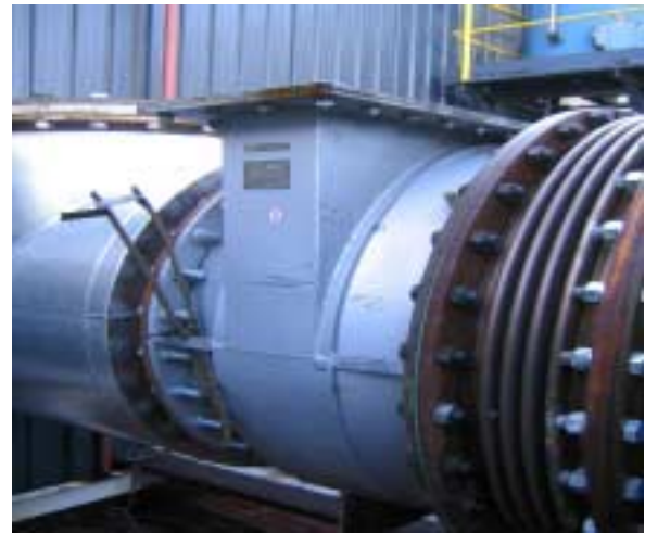
Figure 4: DCL QUICK-LID™ catalyst reactor housing
